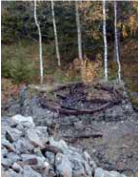
The remains of a turning gear, the point at which the beam drive changed direction.
