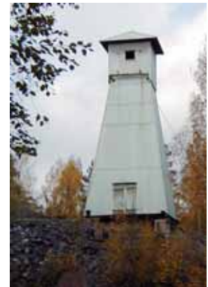
Åker mine's shaft head.
