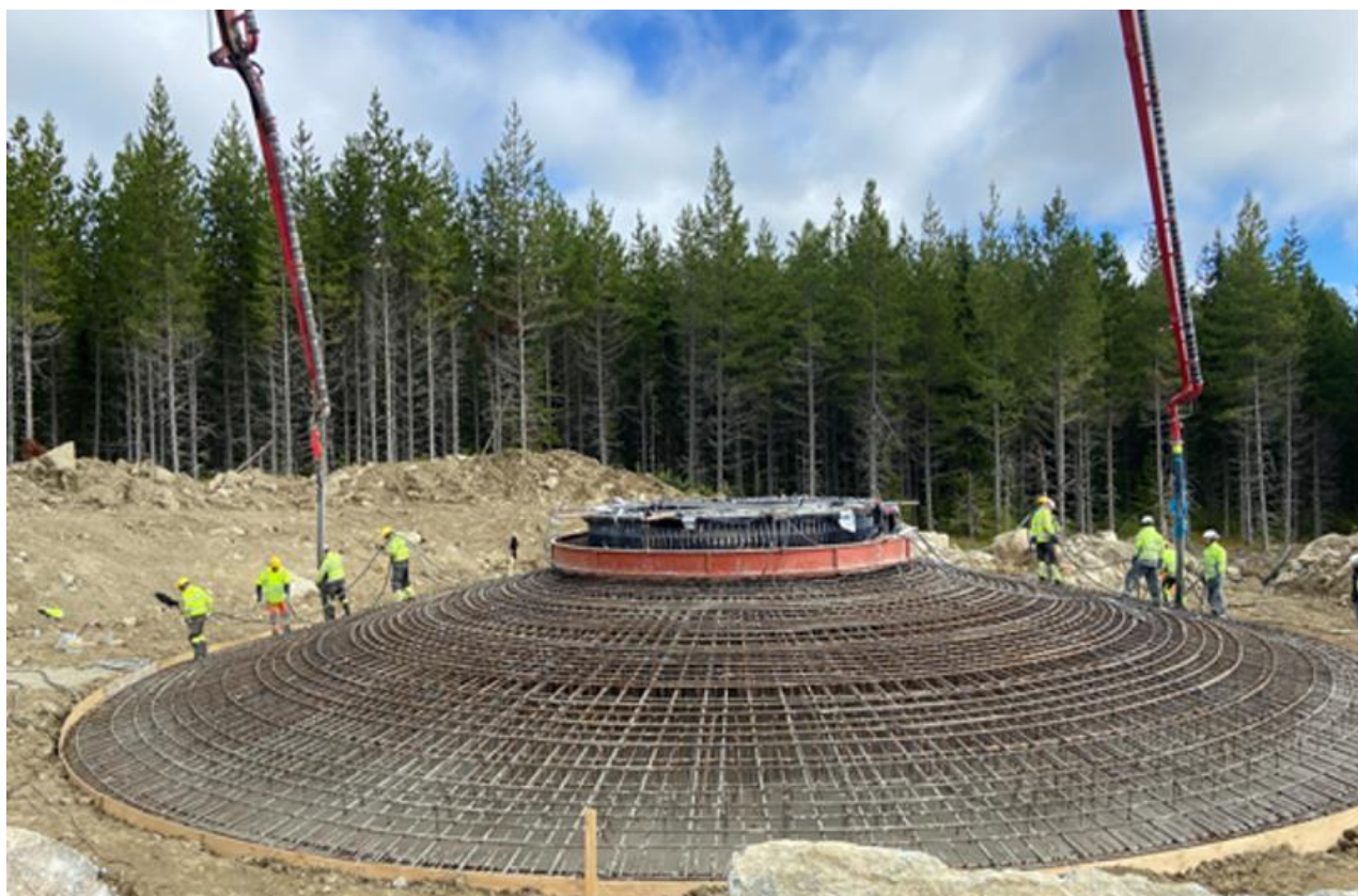
Figur 3 Gravitationsfundament
